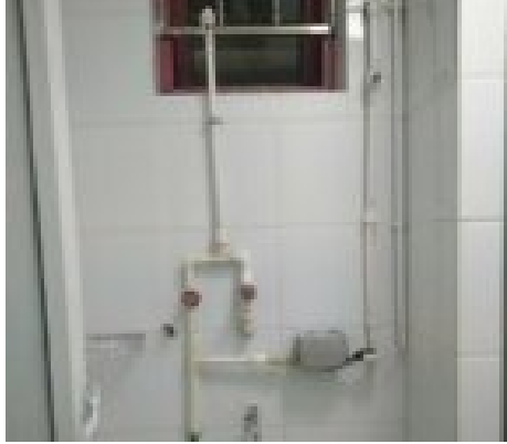
tile fixing bathroom
